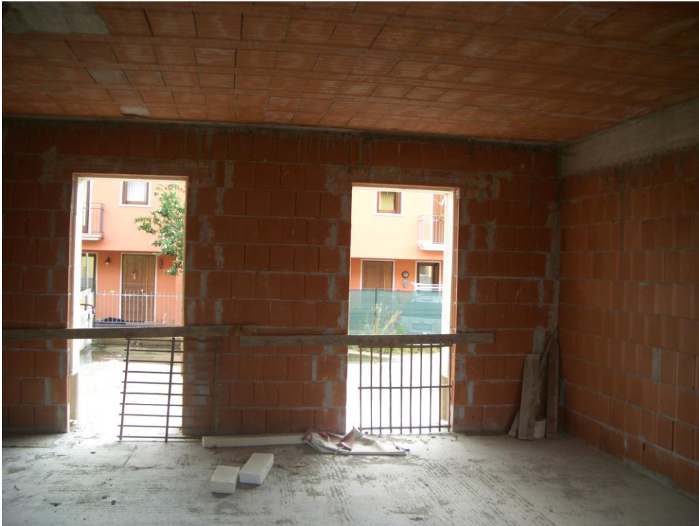
3. Vista interna piano terra
